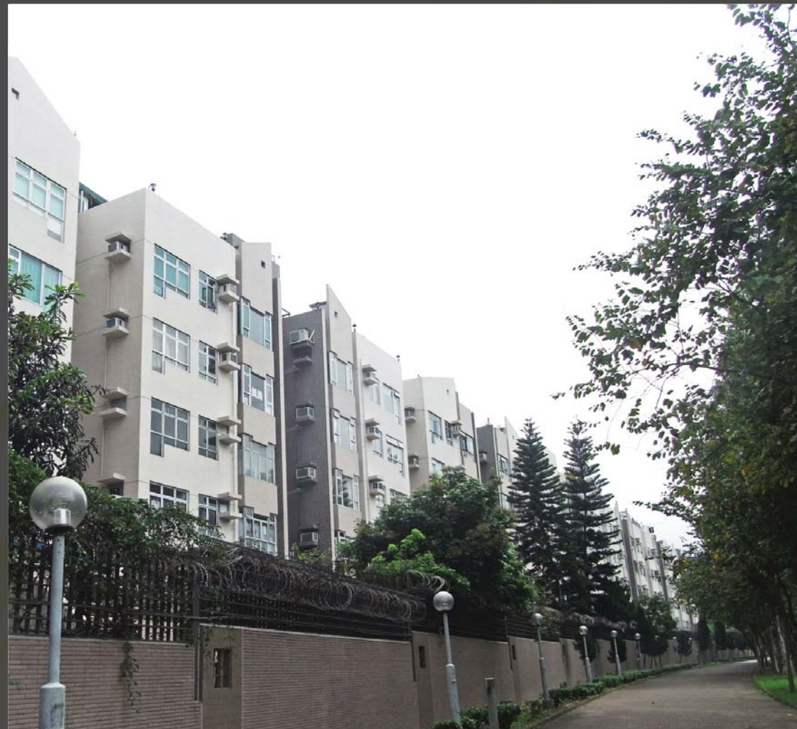
BUILDING RENOVATION WORK FOR TAI PO GARDEN, TAI PO, HK
